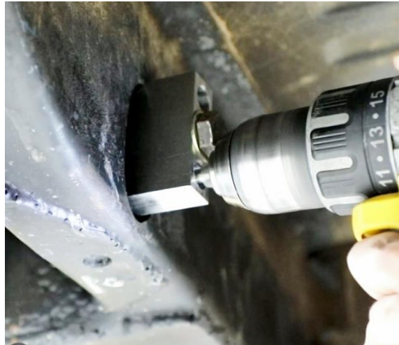
Figure 5 – Drill Pilot Hole
