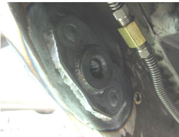
Figure 6 – Inside Doubler and Frame Insert
