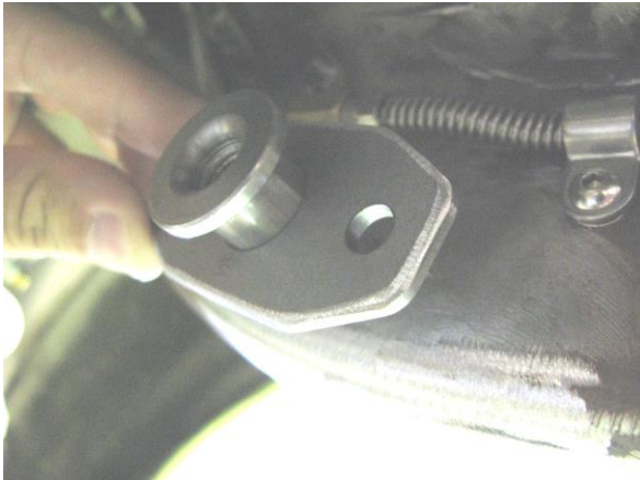
Figure 4 – Locating the Frame Insert and Doubler on the Inside Frame Rail
