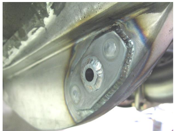
Figure 7 – Outside Doubler and Frame Insert
