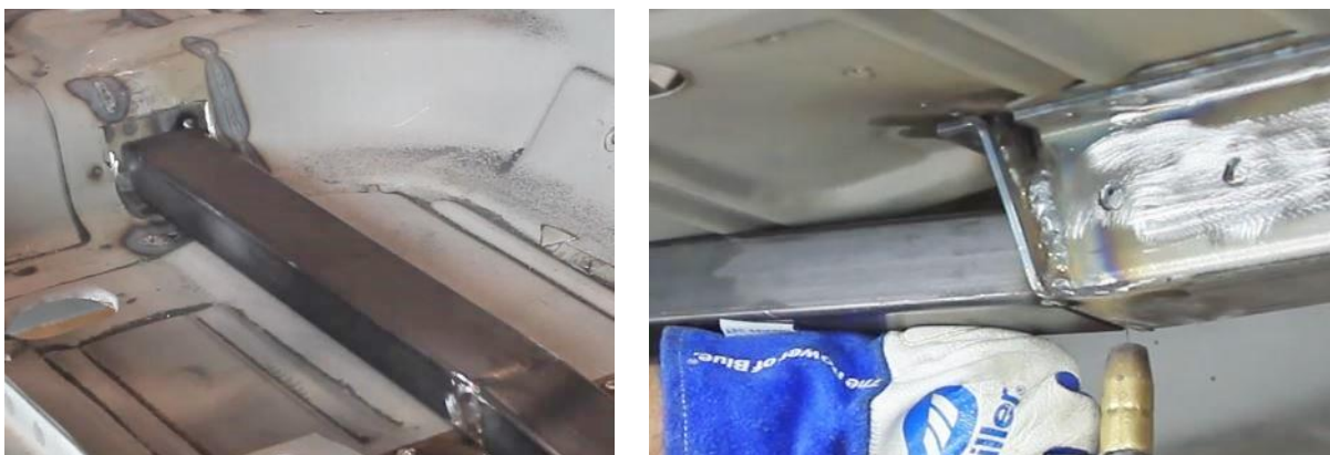
Figure 14 - Tack Weld Connector in Place
