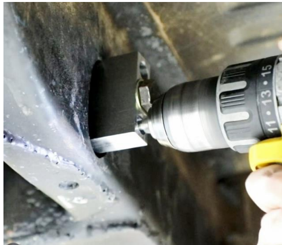
Figure 5 - Drill Pilot Hole
