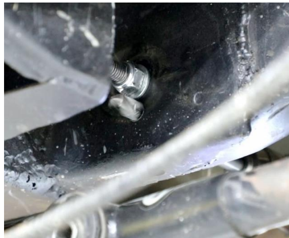
Figure 6 - Drill Bottom Link Hole
