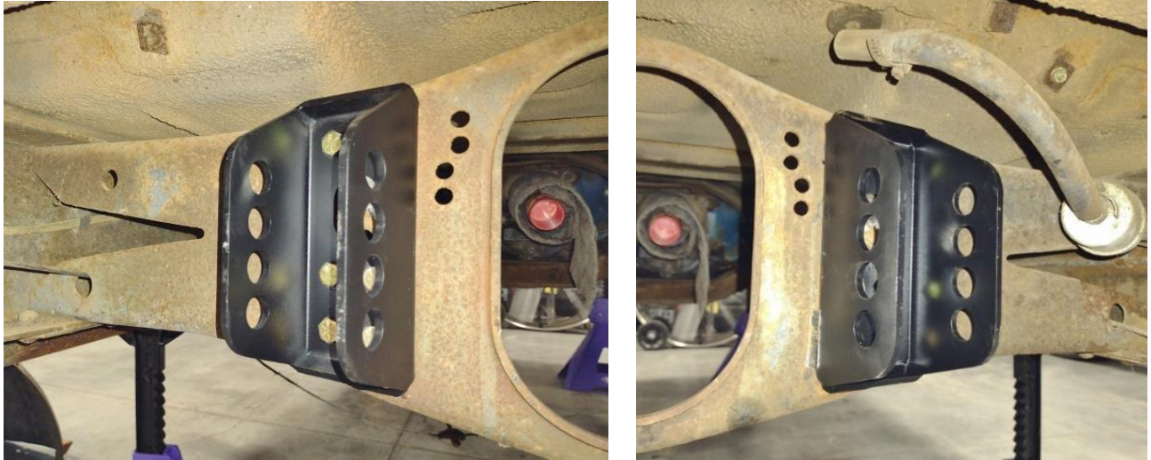
Figure 5 - Install Truck Arm Chassis Mounts
