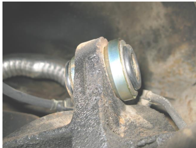
Figure 3 - Replacement Bushing Installed
